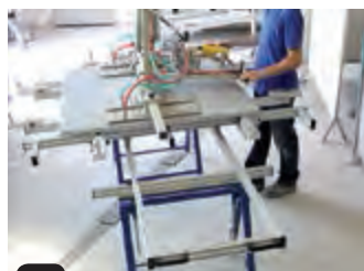
2 loading of slabs
